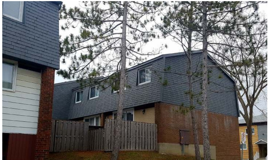
Enviroshingle Installation in Accora Village
